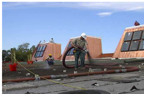
Gregory Scott of Ground EFX applies the growth medium to the Malletts Creek Library Branch on October
