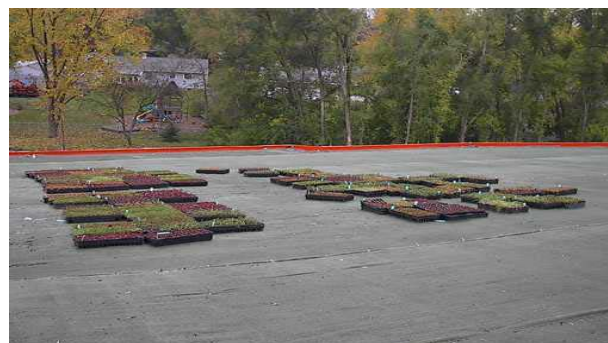
Plugs, in 72-cell trays, wait to be planted on the southeast side of the roof.
